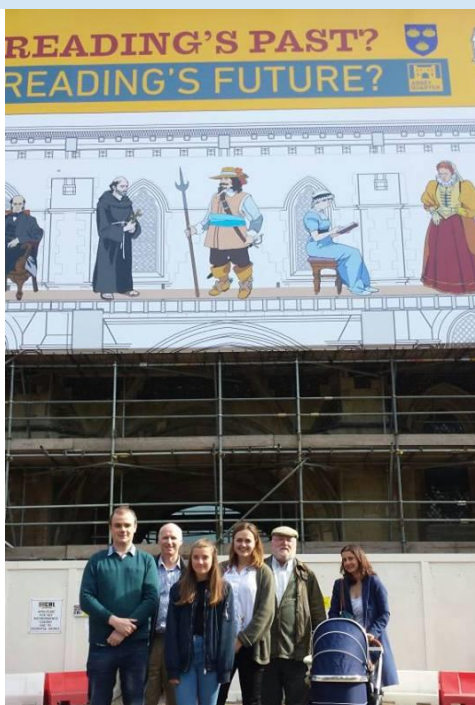
Project staff and volunteers see the new scaffold hoarding for the first time.
