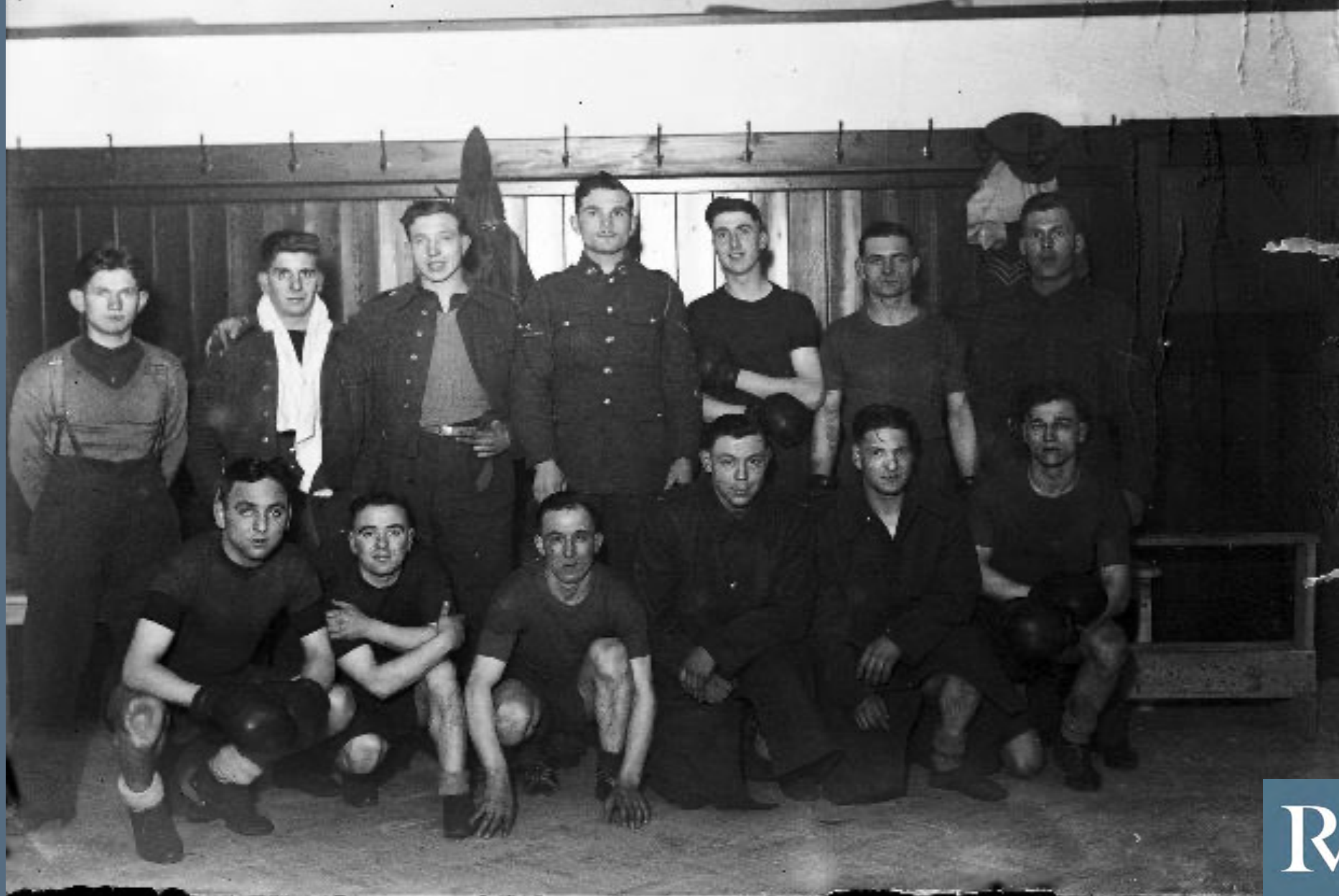
Boxing at Brock Barracks, Reading Photograph from Reading Chronicle Collection - February 1940
